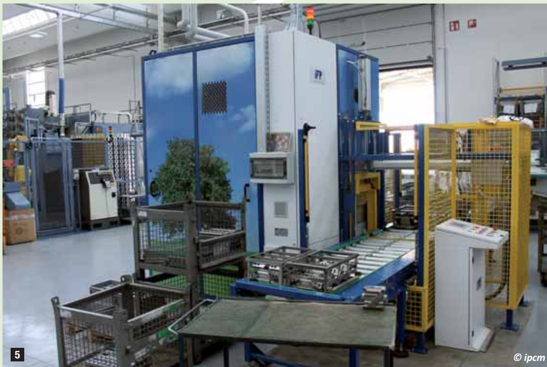
5 The modified alcohols vacuum system installed by IFP Europe in 2013. Within a few months, a second one will be installed, which will cover the entire production needs.
